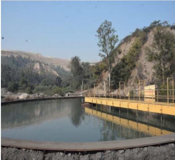
Clarifier of ETP
